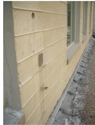
**Figure 23. Testing Site Lightwell Walls After Repair Completion**
