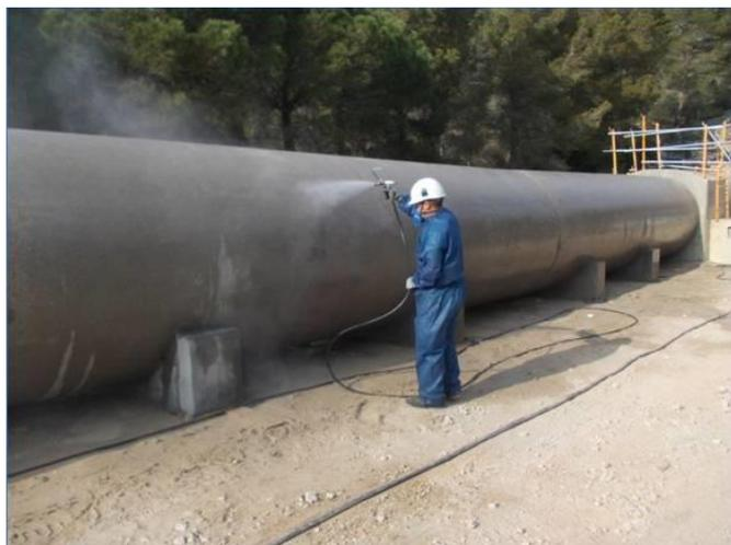
Figure 24. Spraying OCI onto the Pipeline
