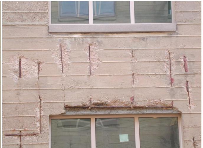
**Figure 19. Example of Corrosion on Lightwell Walls Prior to Repair**
